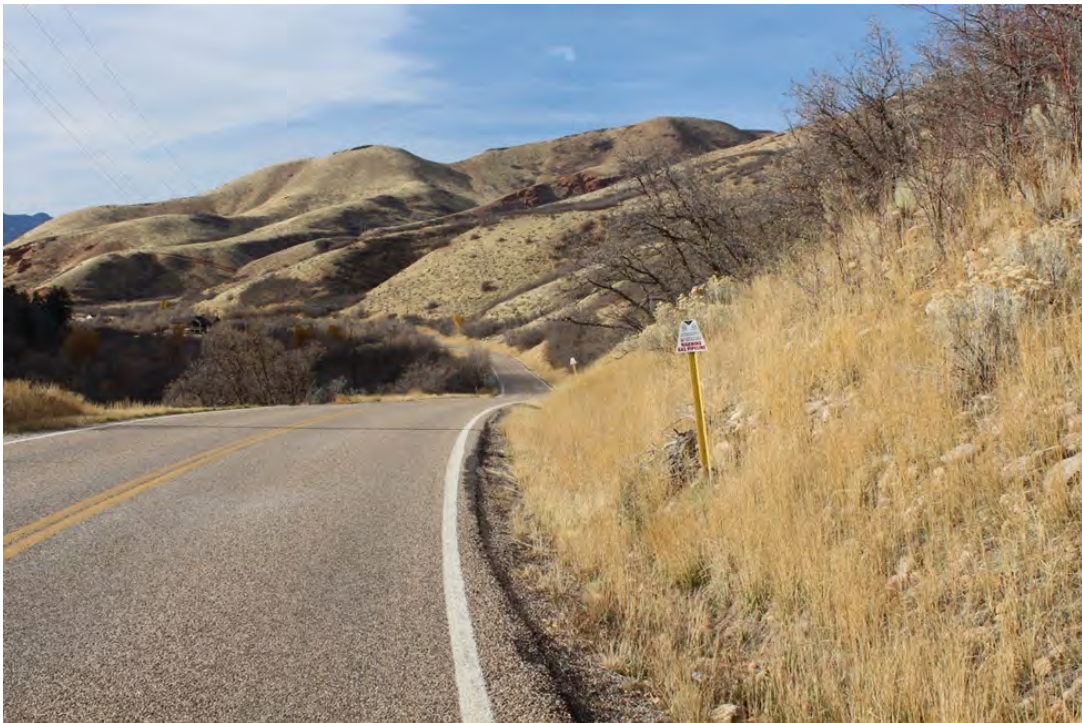
Photo 2.2-2 Example of typical pipeline construction restoration along a roadway.
