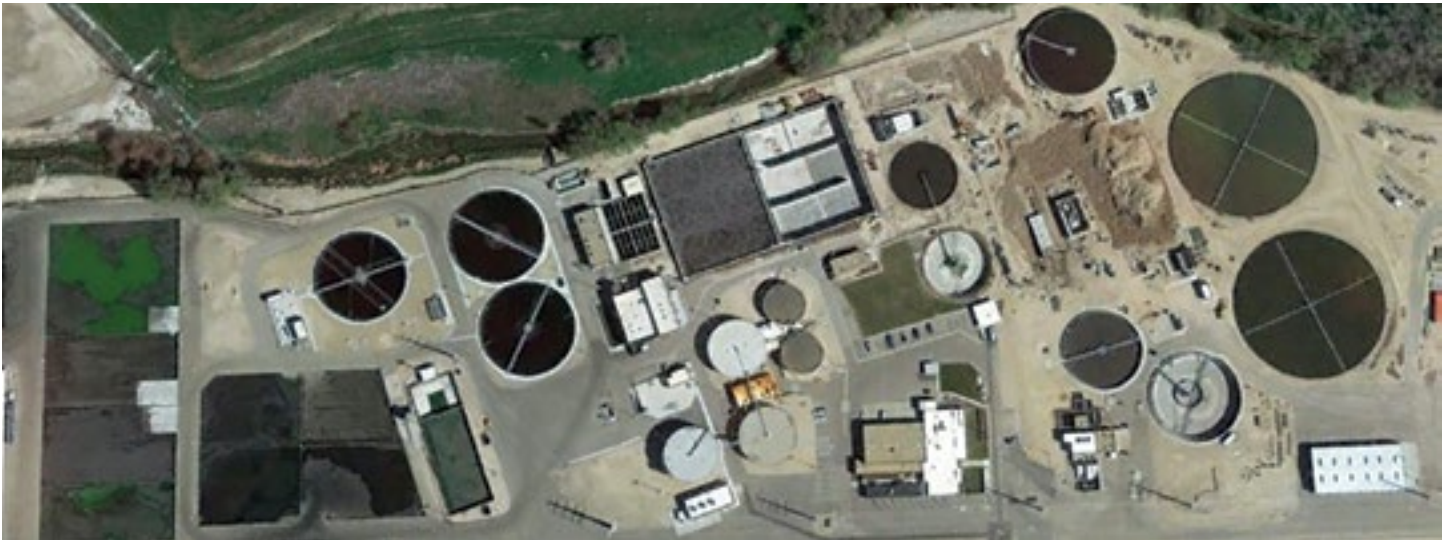
The Nampa wastewater treatment plant is an example of a large facility with mechanical and biological treatment. / Google Earth
