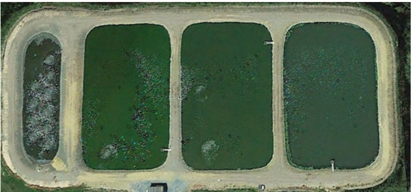
The Inkom wastewater treatment plant is an example of a small lagoon-based facility. / Google Earth
